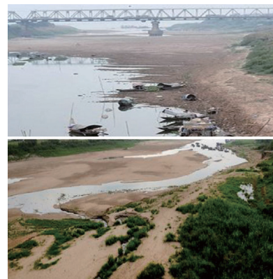
Fig.7 No water flow under a bridge (above) & shoals in the Red River Delta in dry season (below)
