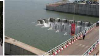
2: Dau_Tieng Dam (Embankment, H30m, W1.5bil.m 3 , Crest Length L1200m,)(left) 3: Phuoc_Hoa Barrage (H28m, Crest Length 400m)(right)
