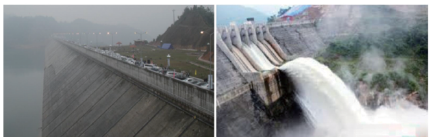
1: Cua_Dat CFRD (H118m, W1.5bil.m 3 , P124MW) 2: Ban_Ve HPP (RCC Dam, H136m, W200mil.m 3 , P230MW)
