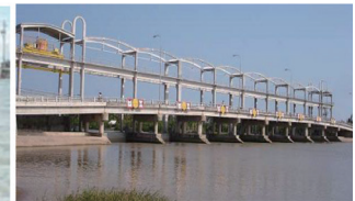
4: Tra_Su Rubber Barrage (Crest Length L400m,)(left) 5: Can_Chong Barrage (H28m, Crest Length 400m)(right)
