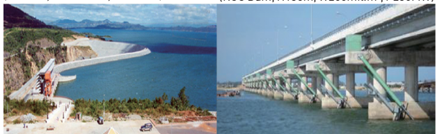
3: Yaly HPP (Rockfill Dam, H69m, W780mil.m 3 , P720MW) 4: Thao_Long Barrage (Crest Length L540m)
