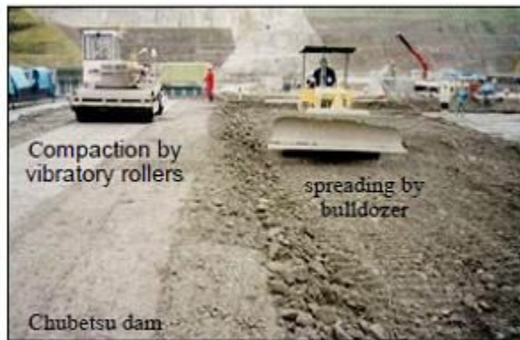
Photo 21- Spreading and compaction in RCD concrete
