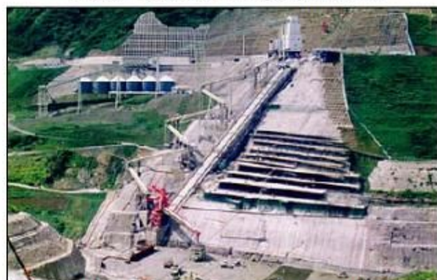
Photo 18 - Belt conveyor, Gassan dam, 1995
