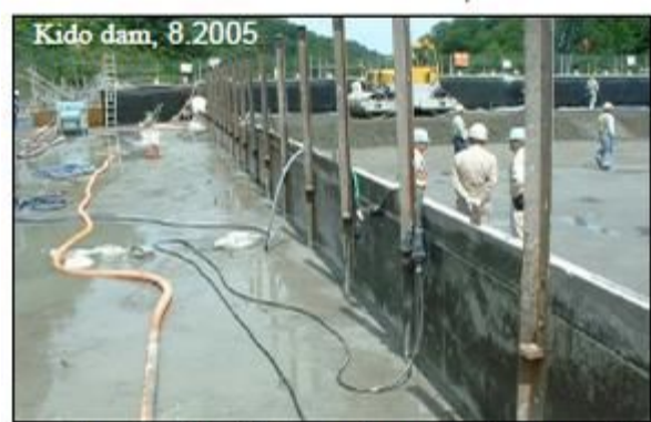
Photo 24- Block forms along the placing end
