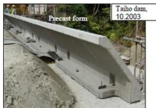
Photo 28- Set up of precast form
