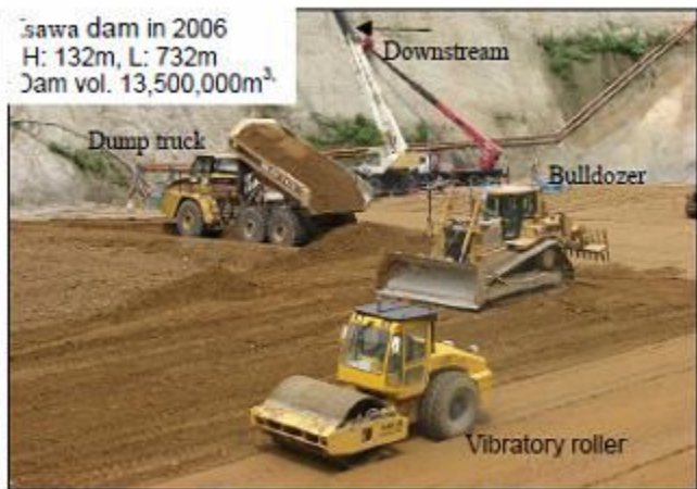
Photo 4 - Mechanized latest rock-fill dam
