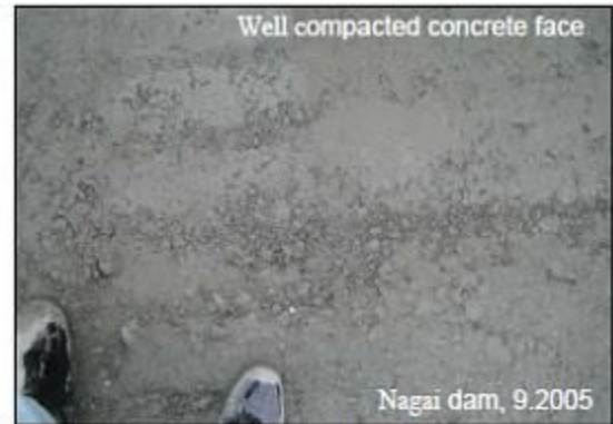
Photo 22- RCD concrete after compaction
