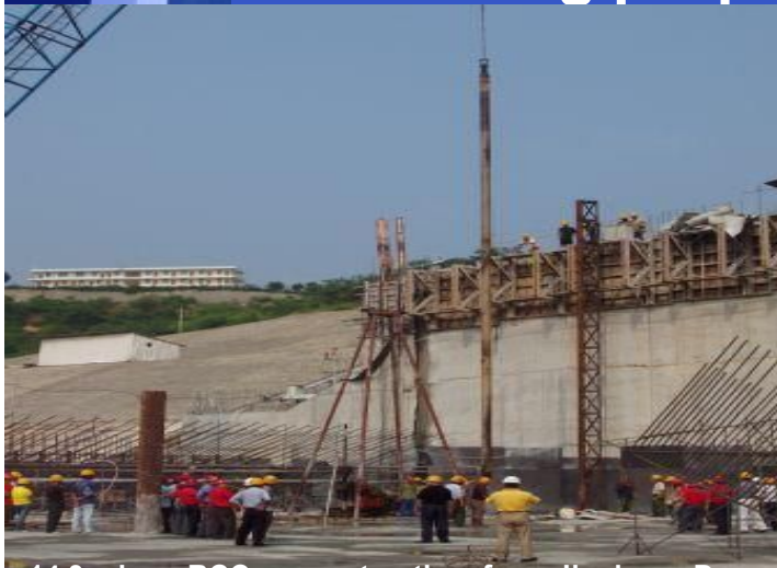
14.3m long RCC core extracting from Jinghong Dam
